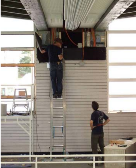
Figure 8: Cameras during installation
